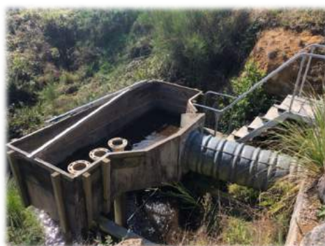
A closer look at the microhydro unit
