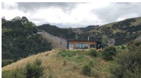
Off-Grid home in Raglan, Aotearoa
