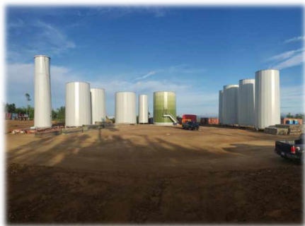
Wocawson Project in early construction. (Photo courtesy of Tanna Pirie)
